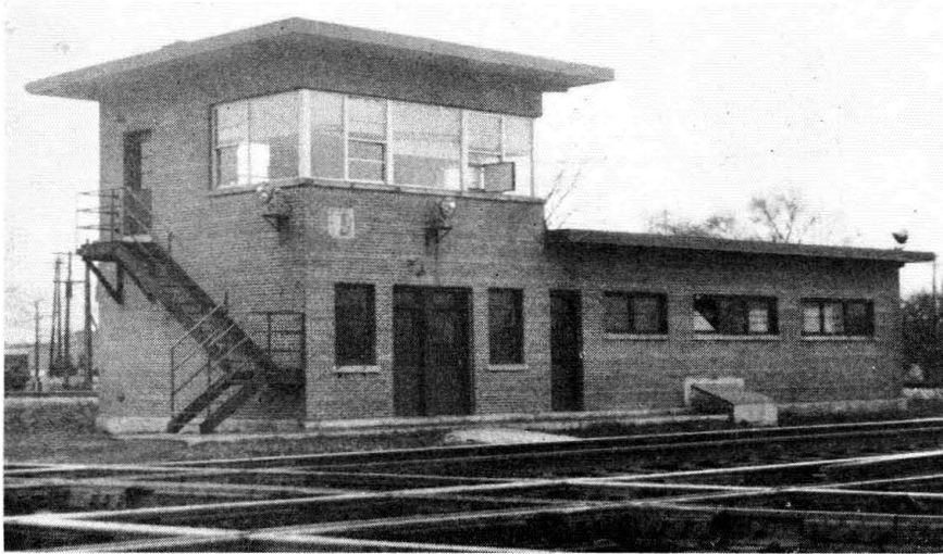
Tower is of fireproof brick, precast-concrete and steel-beam construction
