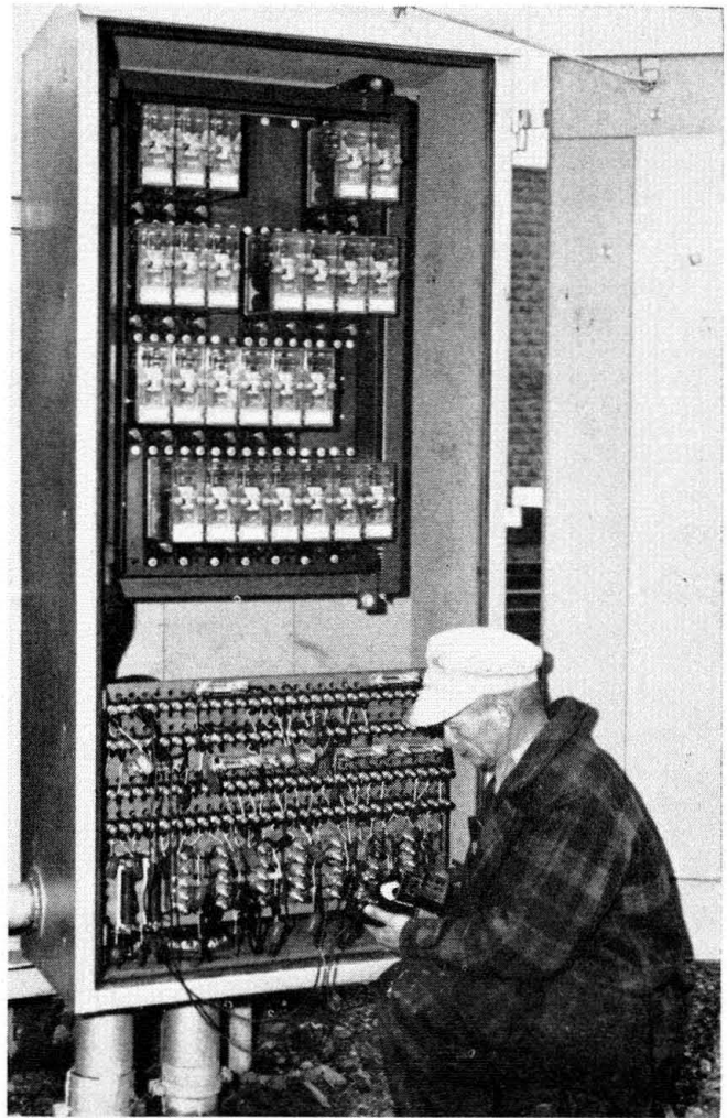
Instrument case, showing terminals and Type-B relays on hinged mounting
