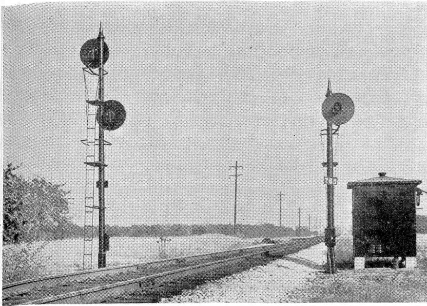
Instrument house at intermediate location
