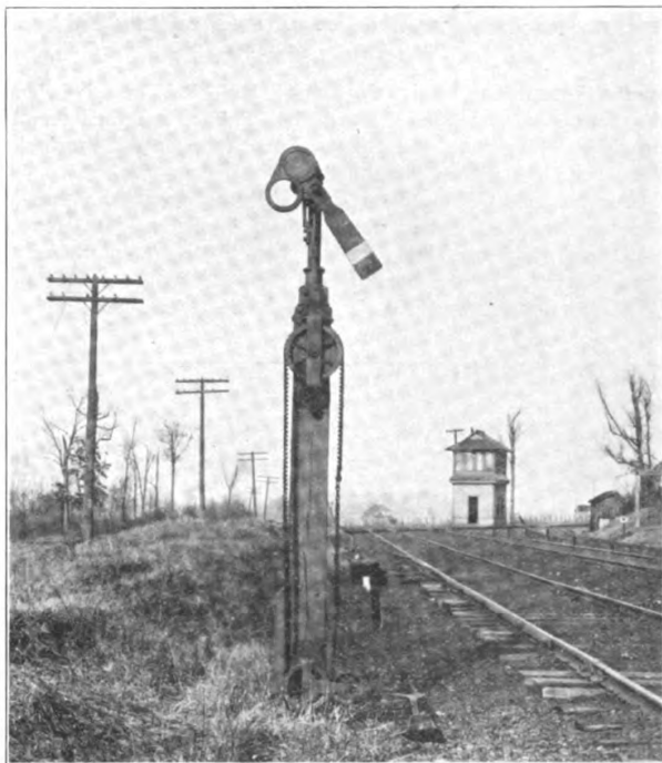
Fig. 1. A Northbound Home Signal at a Side Track. Showing the Method of Operation, Wire Connection, Etc.
