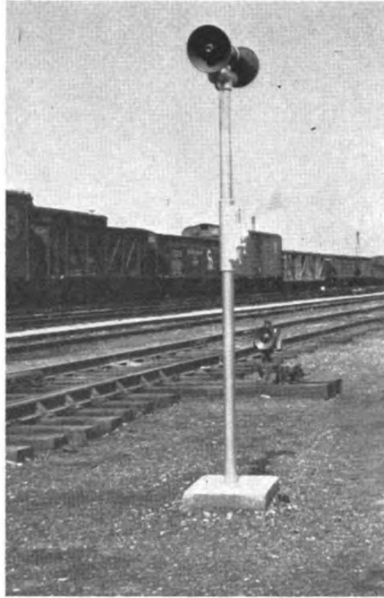
Typical talk-back loudspeaker mounting
