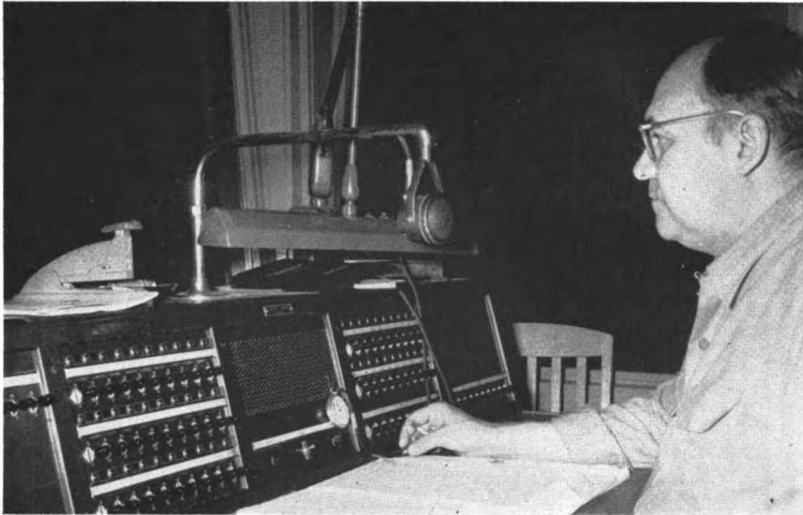
Yardmaster is able to talk to men in yard via 48 talk-back and 21 paging loudspeakers
