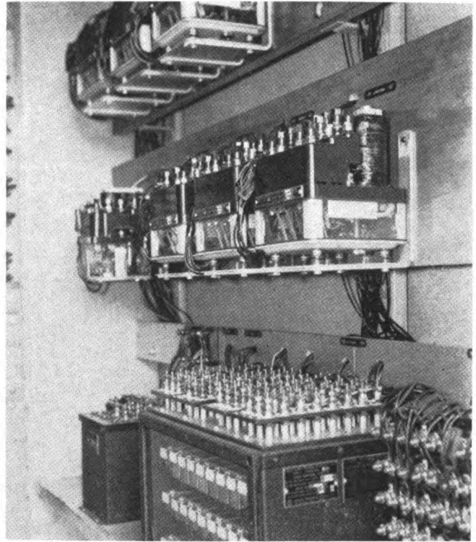
The relays are equipped with plug couplers
