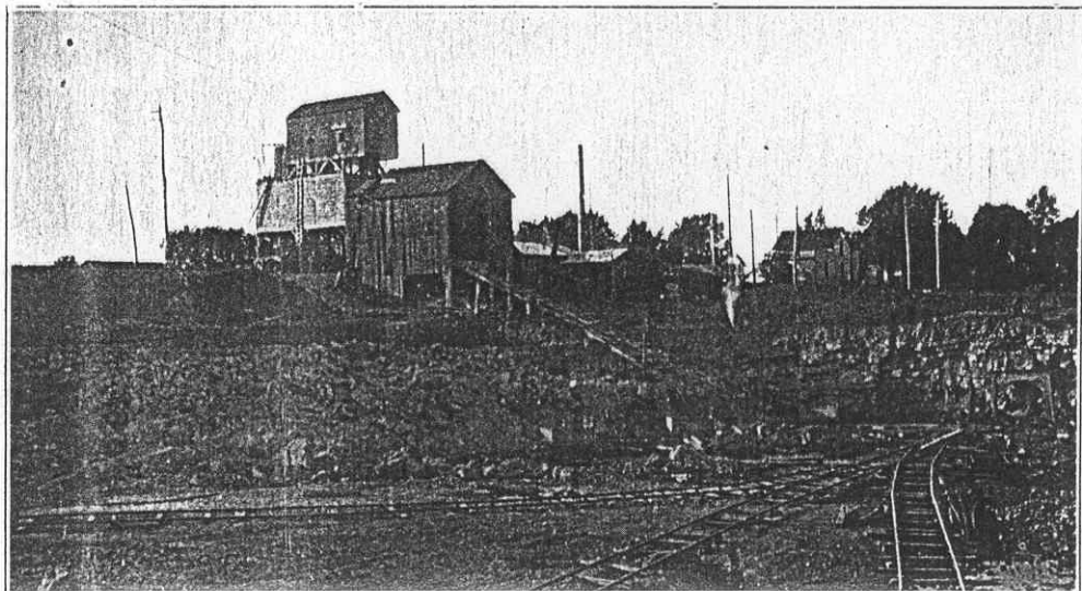
THE QUARRY AND STONE-CRUSHER PLANT AT NEWPORT, OPERATED BY THE RAILROAD COMPANY, FROM WHICH 60,000 CU. YDS. OF STONE BALLAST HAS BEEN REMOVED FOR TRACK BALLASTING
