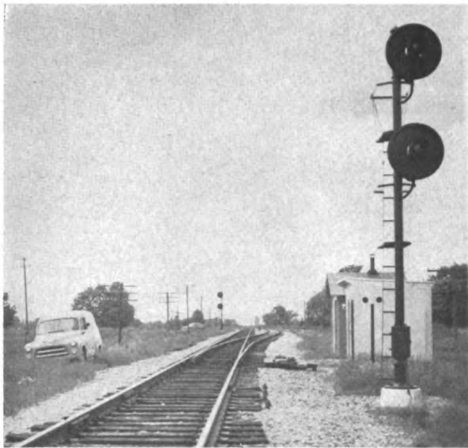
POWER SWITCH layouts are well constructed
