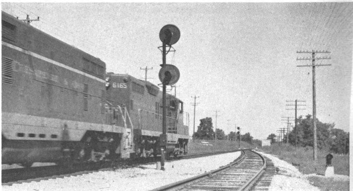
Siding thrown over to locate main track signal between main and siding
